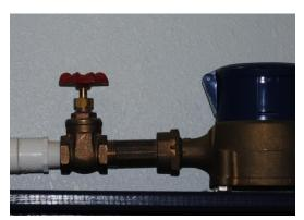
Shut-off valve needs to be installed right after meter.
